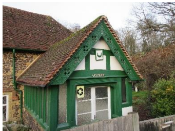
Two other examples of local bargeboard detail
