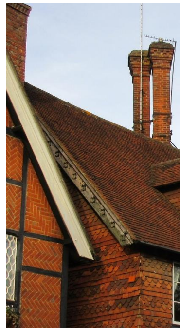
Above: the Old Post Office, bargeboard detail
