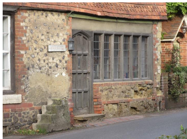
Chalky stone and flint, trimmed with brick
